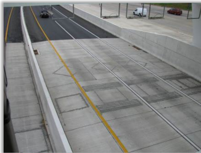
Figure 2-6: Example of an Axle-Based Automatic Vehicle Detection and Classification Loop Layout Installation
