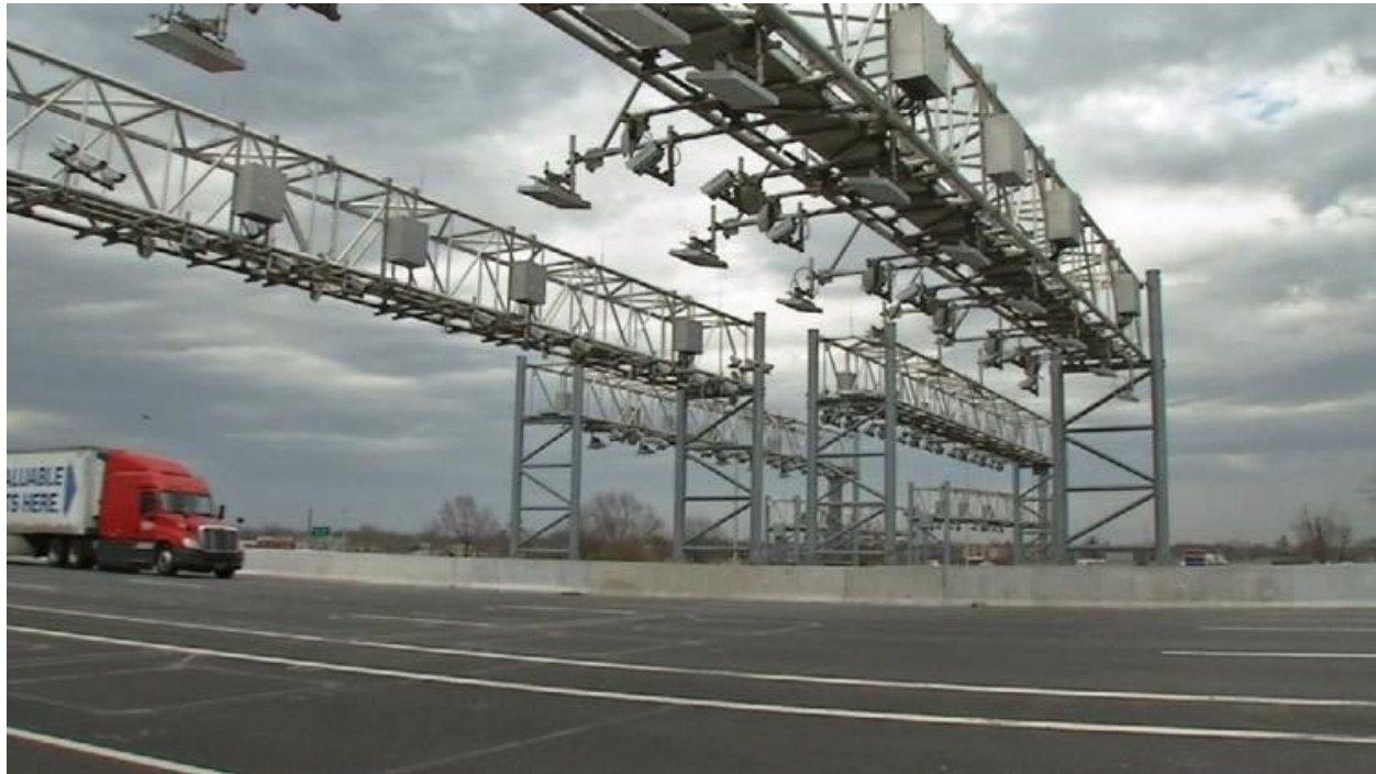
Figure 2-3: Toll Gantries (Ohio River Bridges)
