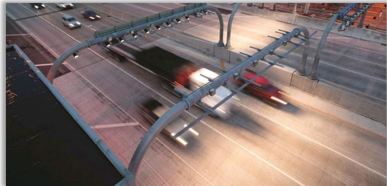
Figure 2-1: Example of an All-Electronic Tolling System Toll Zone
