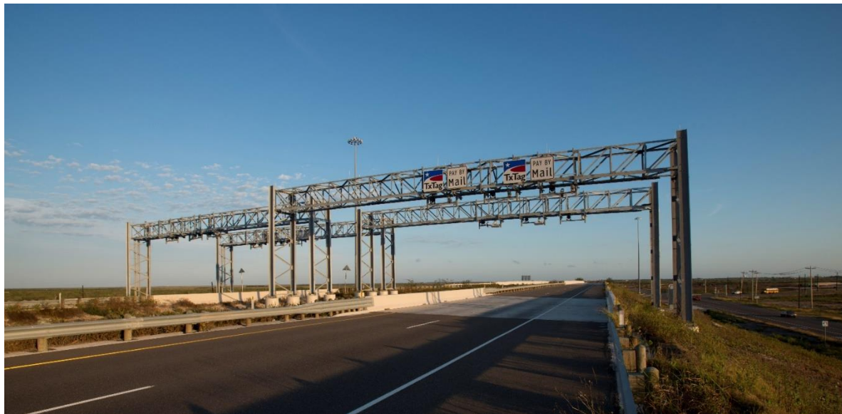
Figure 6: Example of a Set of All Electronic Tolling Gantries
